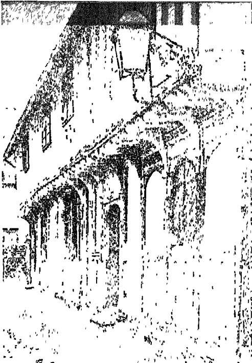
§ 152 Tudor cottages, Chiddingstone, Kent Note the use of brick between the timber uprights
